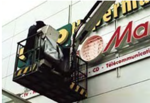
Fig. 2: Sign electricians work on high-voltage circuits -- which are sometimes energized -- in awkward locations. Shown here is an electrician working from a 160-ft. elevation, bucket truck
